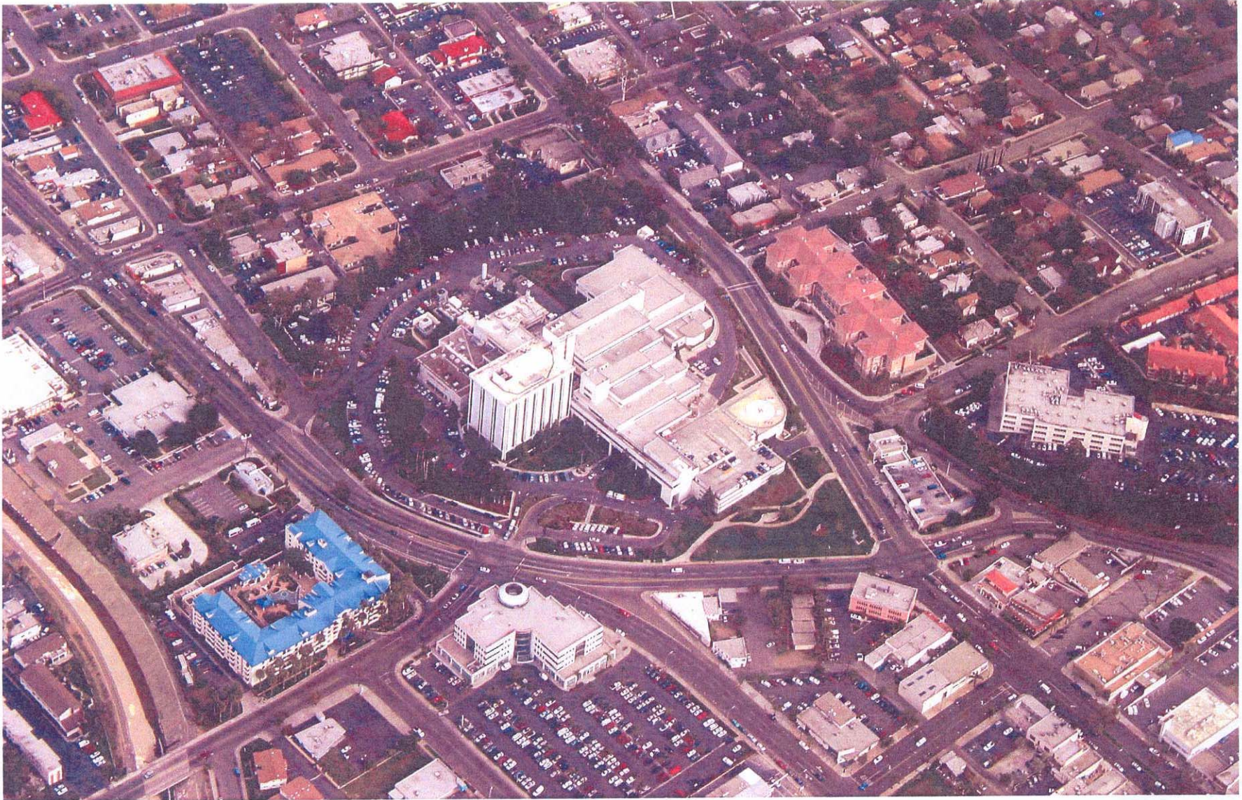
Photo 1-1 Aerial View of Palomar Medical Center
